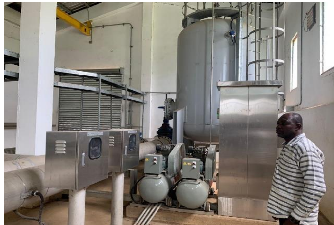
Rehabilitated non- return valves at Headworks – UWR
