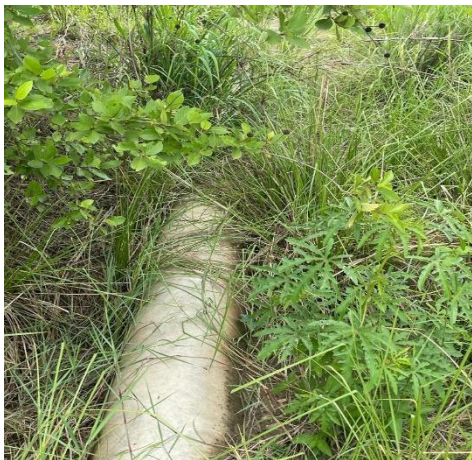
Portions of rehabilitated Transmission pipeline at Salaga
