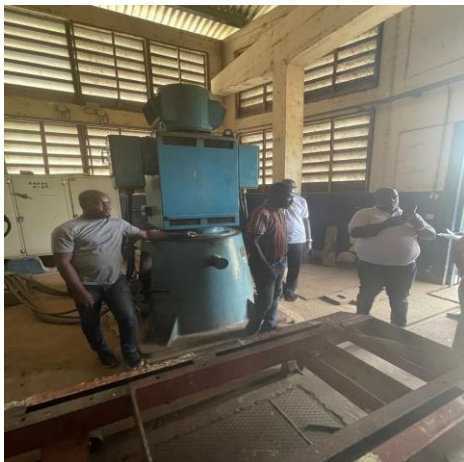
Rehabilitated pump at the Dalun intake, Tamale
