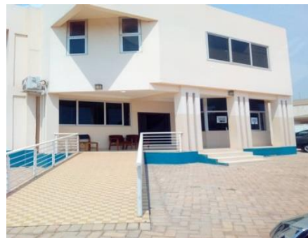
Figure 16: Newly constructed office of GWCL
